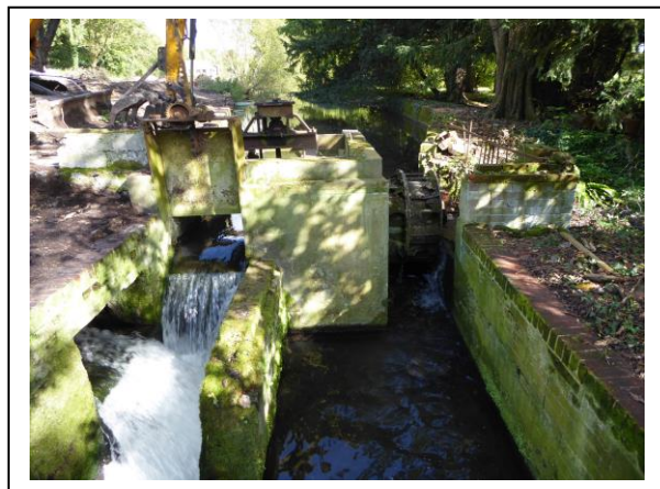
Structures at the weir scheduled for demolition
