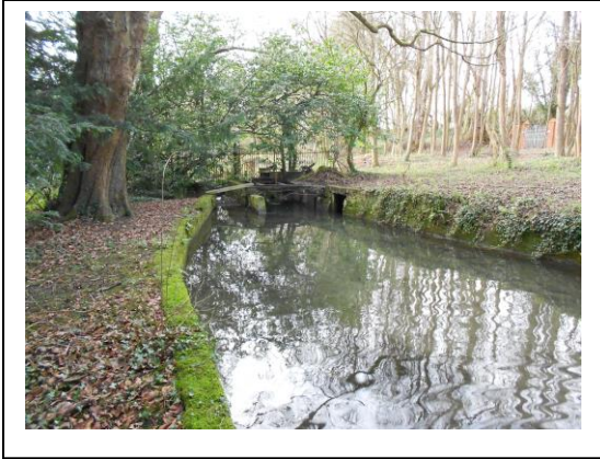
The mill pond above the weir, 2016
